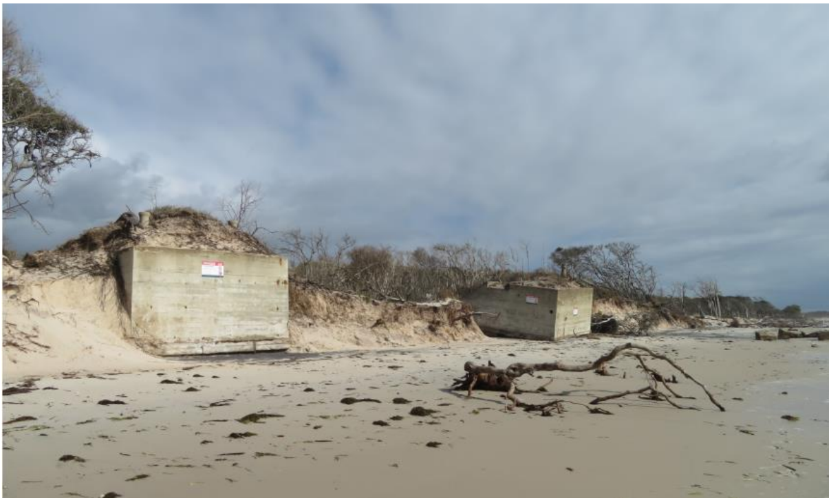
Mine Control Rooms. Photo March 2019, Leanne Siebuhr © Qld Govt.
