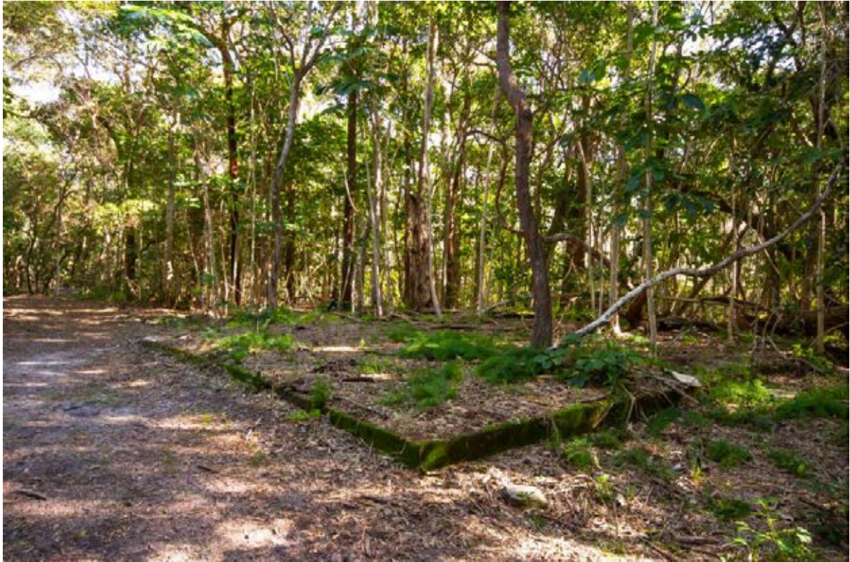
Sleeping quarters footings. July 2018, Matthew Nash-Arnold © Qld Govt.
