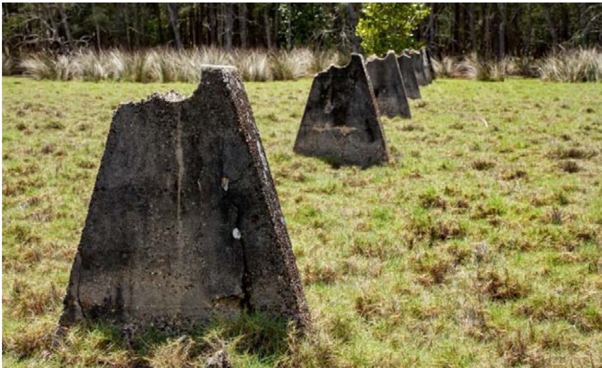
Septic line piers, looking east to the septic tank. November 2018, Matthew Nash-Arnold © Qld Govt
