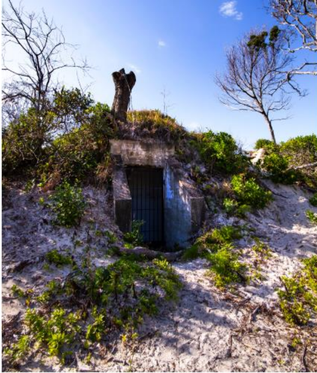
Mine Control Room entrance. Photo July 2018, Matthew Nash-Arnold © Qld Govt.
