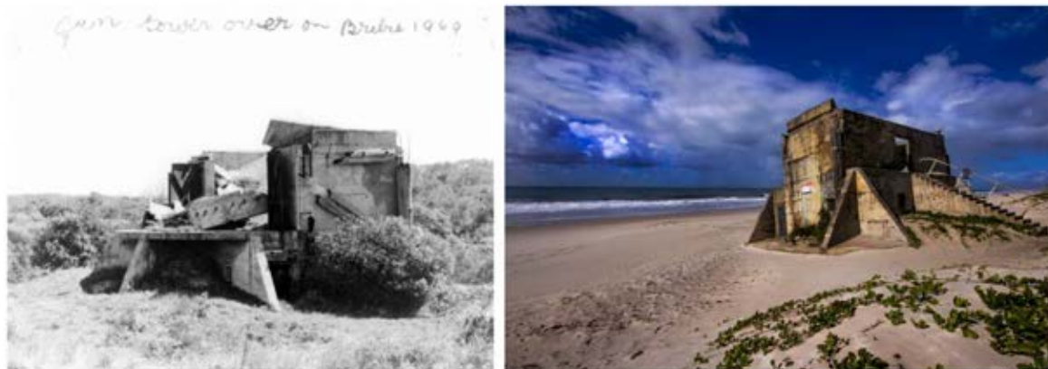
Northern gun emplacement — 1969, left, (© Sunshine Coast Libraries) and 2018, right, (Matthew Nash-Arnold © Qld Govt). The photographs demonstrate the significant beach erosion impacting the structure.
