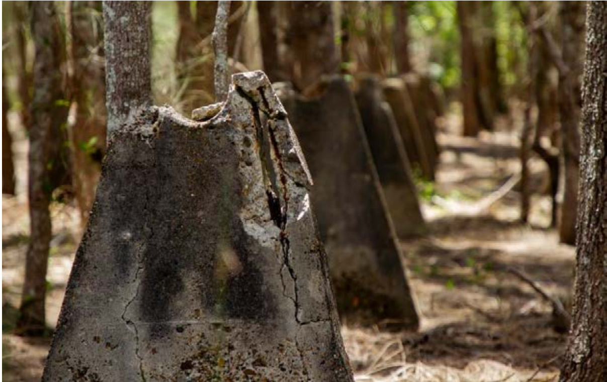
Septic line piers. November 2018, Matthew Nash-Arnold © Qld Govt.
