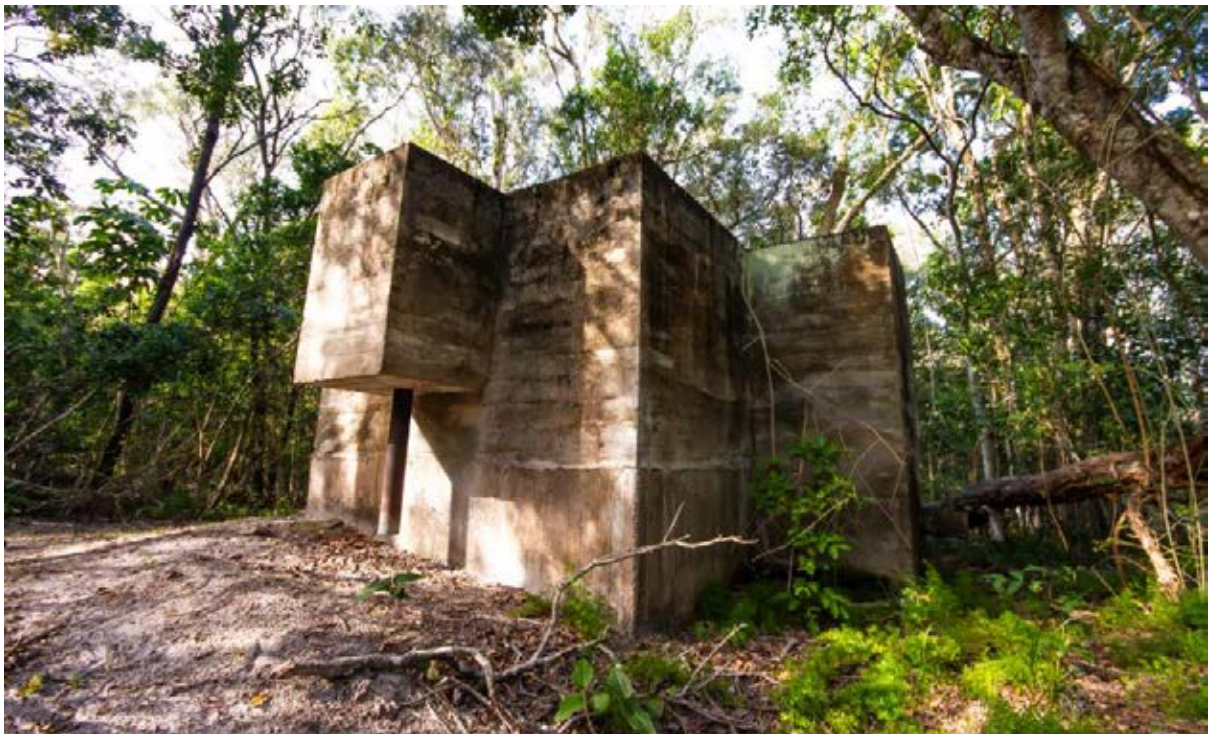
Septic tank. July 2018, Matthew Nash-Arnold © Qld Govt.
