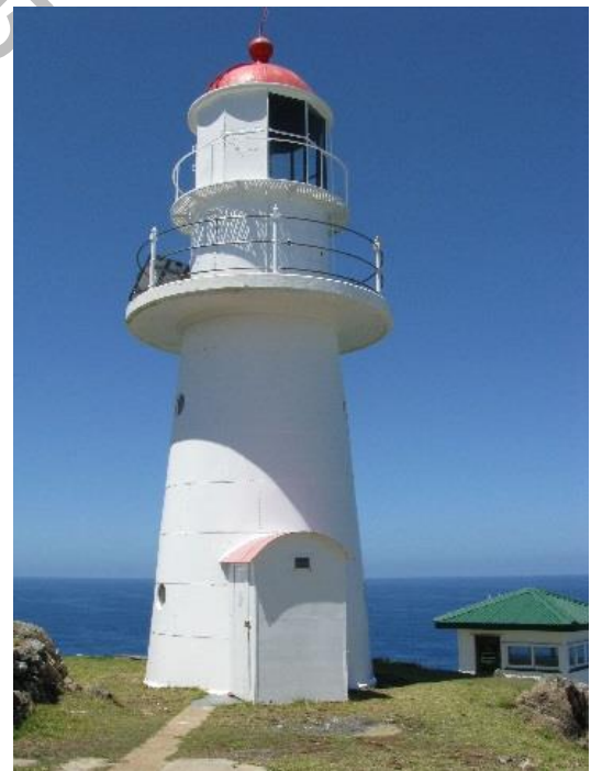
Figure 12. Double Island Point Lighthouse © Queensland Heritage Register
