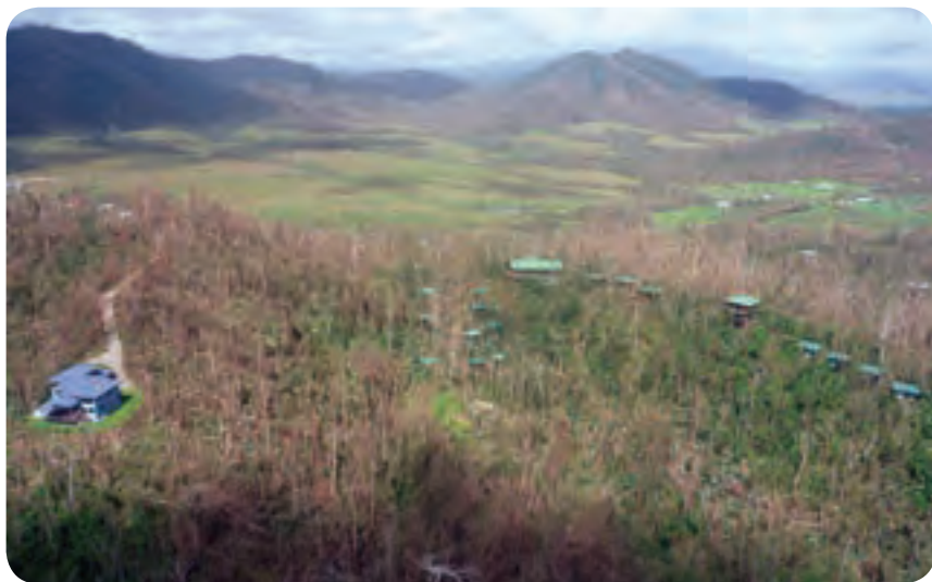
Be aware of changed fuel conditions next to assets and infrastructure after cyclonic wind impact. Audrey Reilly, QPWS, Cyclone Yasi, Bingal Bay (2011).
