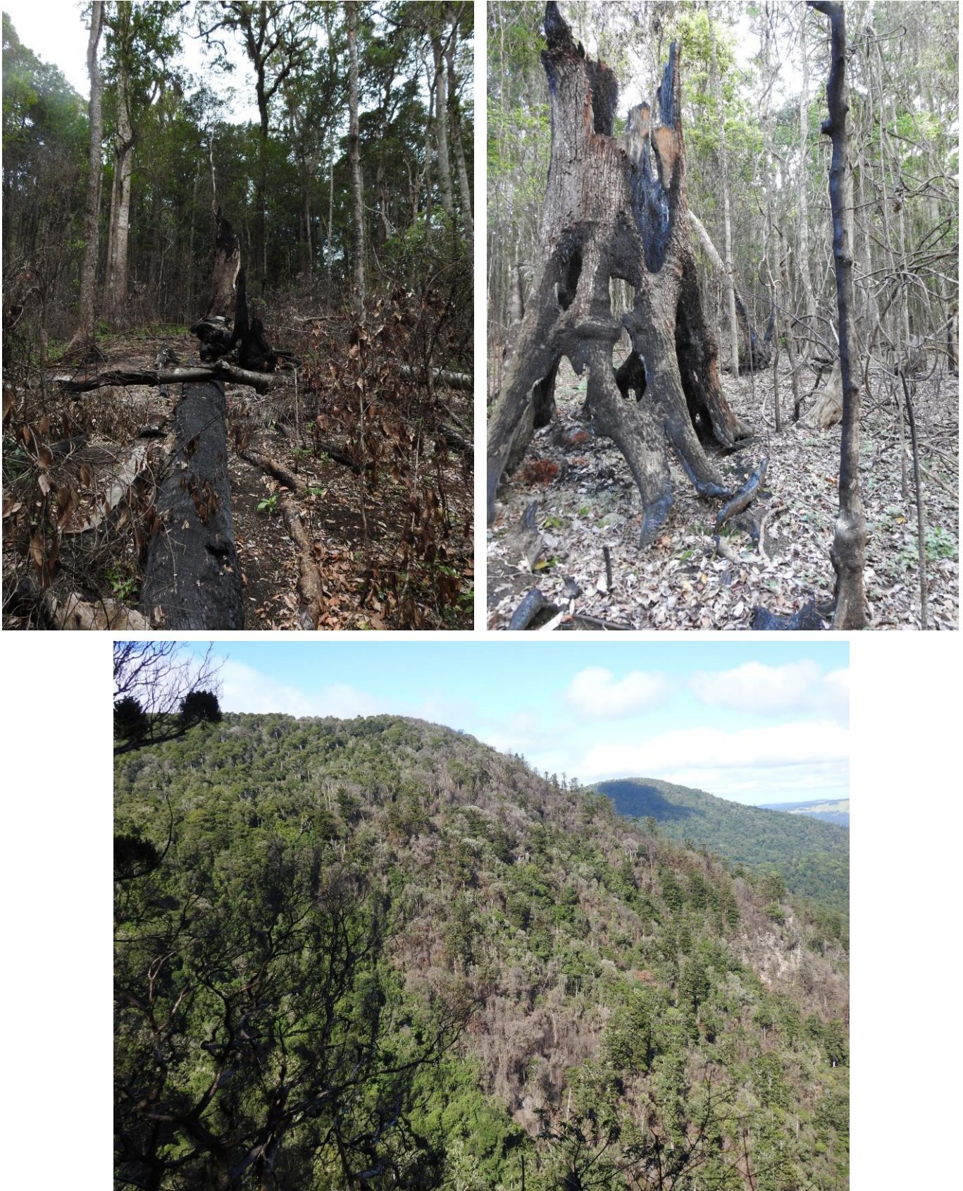
Figure A1.4. Impacts of the fire on upland complex notophyll vine forest at Main Range NP.
