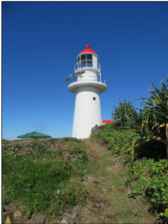
Figure 11: View to lightstation tower from path off concrete track on the north side of the cottages clearing. View to SE (Converge 2020).
