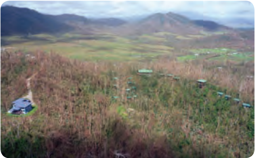
Be aware of changed fuel conditions next to assets and infrastructure after cyclonic wind impact. Audrey Reilly, QPWS, Cyclone Yasi, Bingal Bay (2011).
