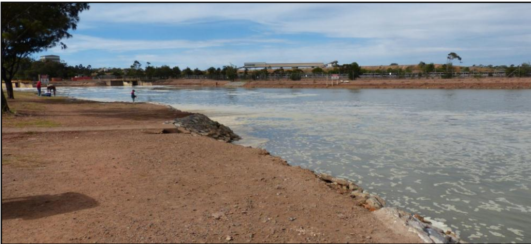
Figure 9.2: NRG Power Station hot water outlet
