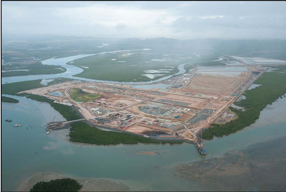
Figure 9.3: Wiggins Island Coal Export Terminal construction
